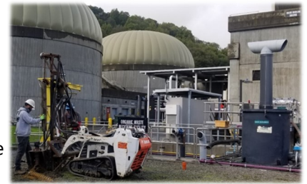
Geotechnical boring for new above-grade storage tank location.
