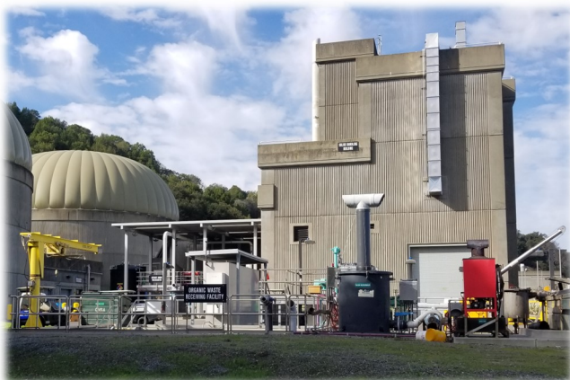
CMSA Organic Waste Receiving Facility
