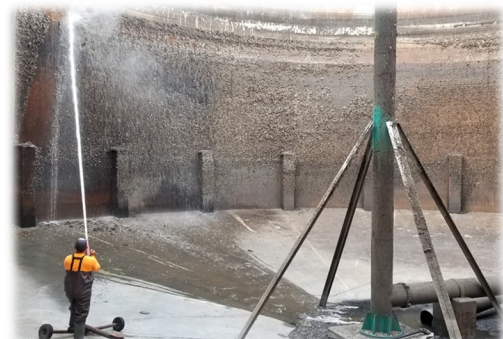
Cleaning wall deposits inside Digester No. 2.
