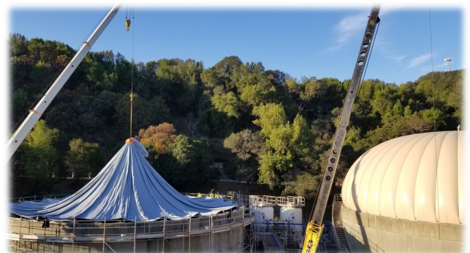
Digester No. 2 cover replacement.
