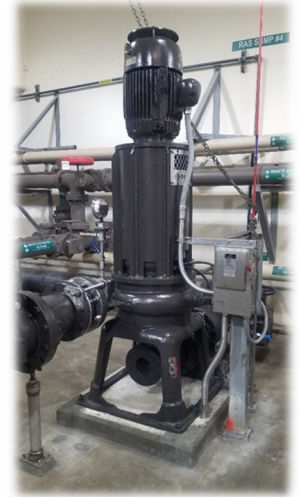
RAS pump after replacement.
